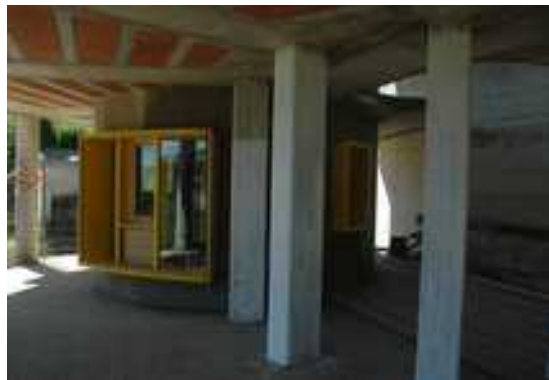
Photo 6: The multi-purpose space built with wattle-and-daub and light earth and grafted into an abandoned concrete-skeleton in Casaprota, Italy
