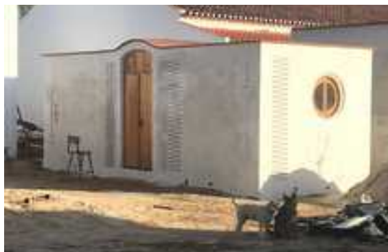
Photo 3: The artist's residence built in Montemor-o-Novo, Portugal during the course on compressed earth blocks
