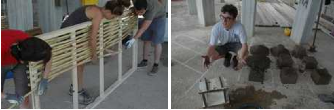
Photo 4+5: Participants assembling Quincha-frames and practical exercises to assess quality of local earth
