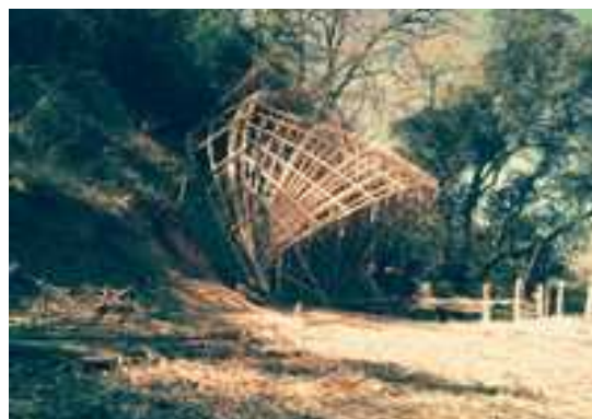
Photo 12: The cane canopy for outdoor lessons in Colleserola, Spain before being covered.
