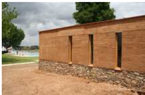
Photo 15: The rammed earth library near the municipal swimming pool in Valverde de Burguillos, Spain
