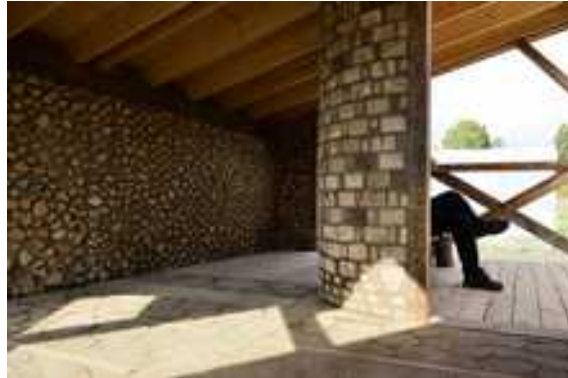
Photo 9: Inner view of the boutique for Östertälje's farmer cooperative in Sweden, built with cordwood.
