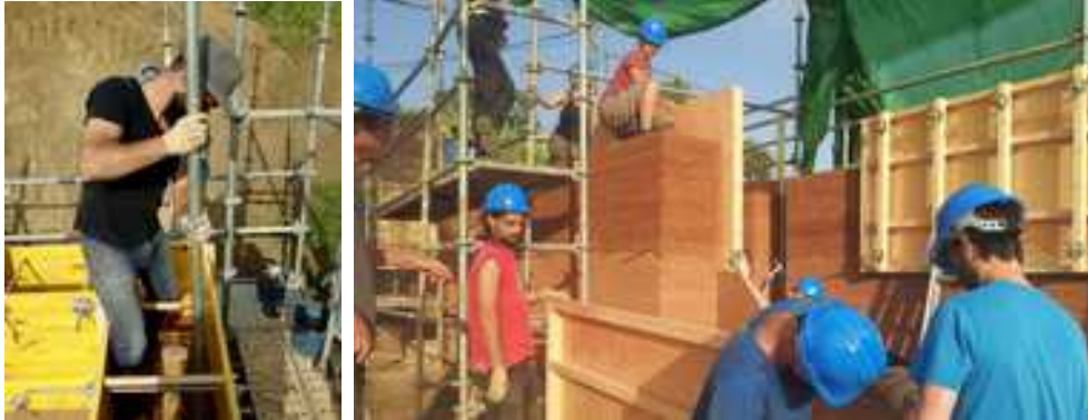
Photo 13 + 14: Manual ramming and collaboration between trainees and experts while removing formwork.
