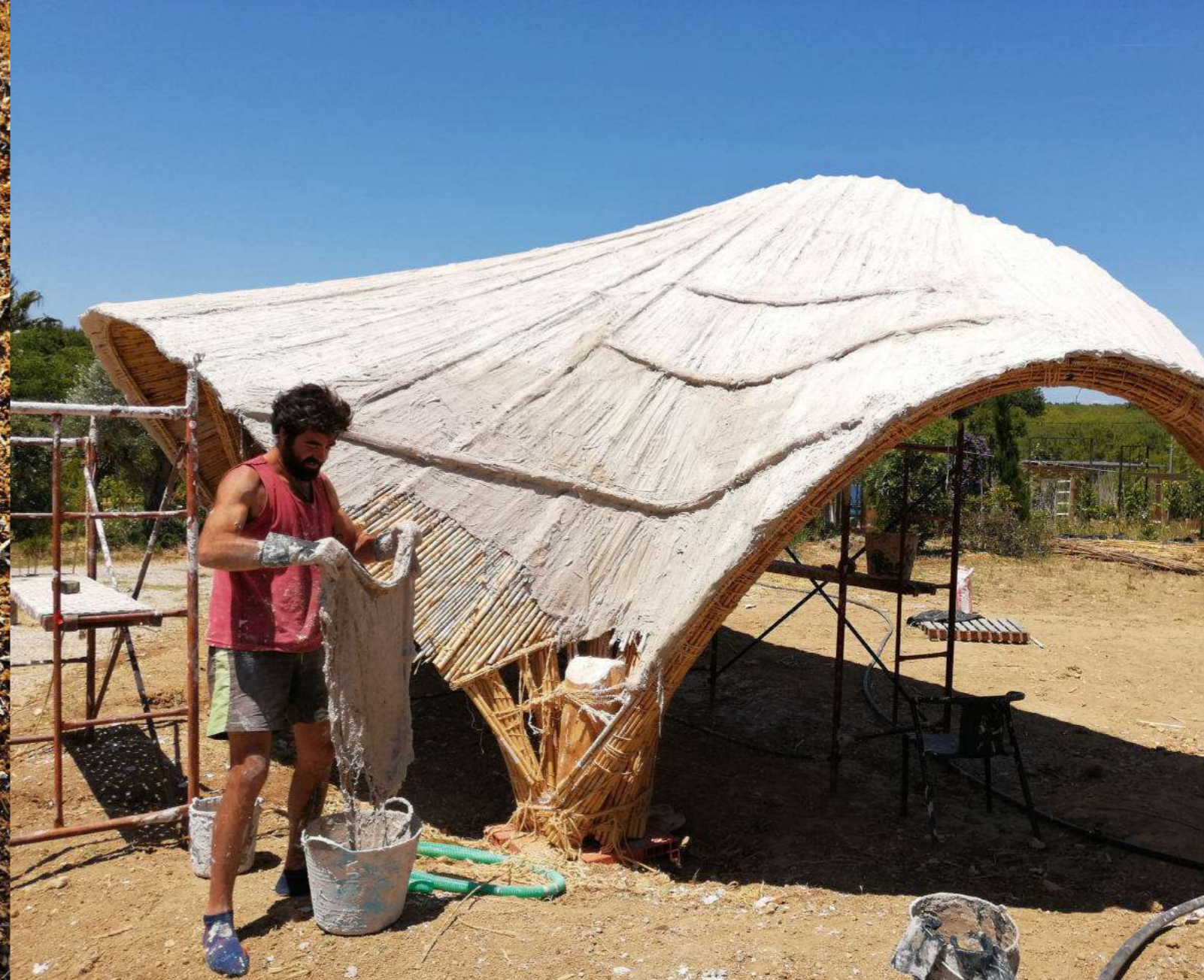
First layer: gypsum being applied with hessian cloth
