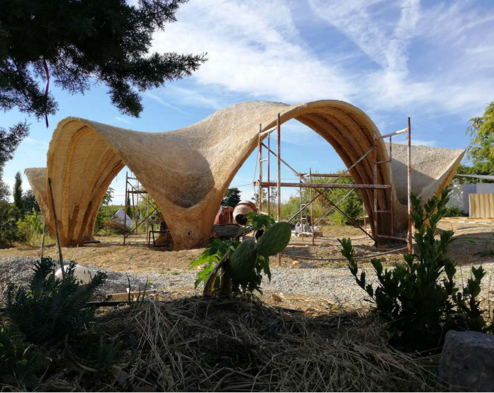
Layer of gypsum with shredded cane on the entire structure
